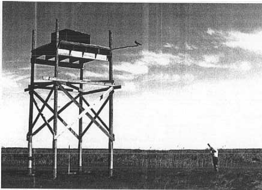
Figure 11. Standard four-pole nesting tower, Sedge Island, New Jersey Note metal predator guards.
