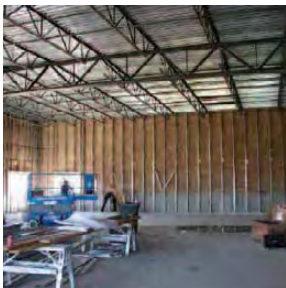
2006 was the "year of construction" for TAF.
