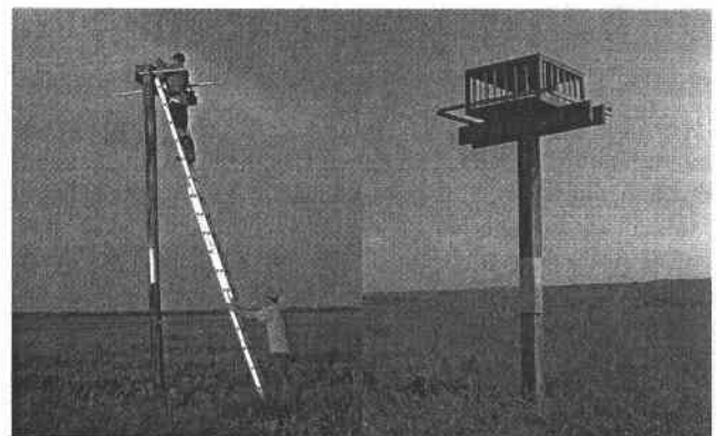
FIG. 1. Two designs of artificial nests provided for Aplomado Falcons in southern Texas. The “platform” design on the left is an open platform mounted on a 6-m pole; the “barred” design on the right is a solid-topped box with conduit sides spaced to allow birds access to the nest, mounted on a 3.5-m pole.
